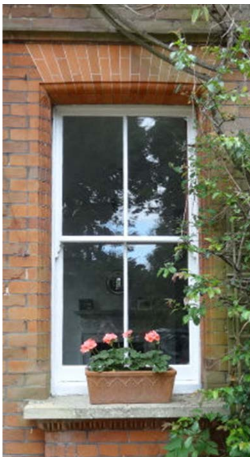
Window at Howdah with rubbed brick head and sill
