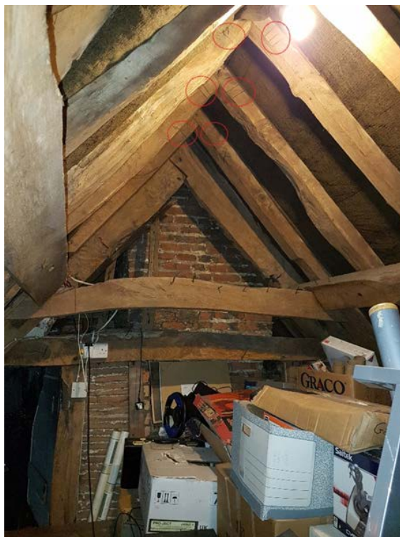
Open roof in attic floor with hip end, carpenters' marks (I. II and III) and chimney.
