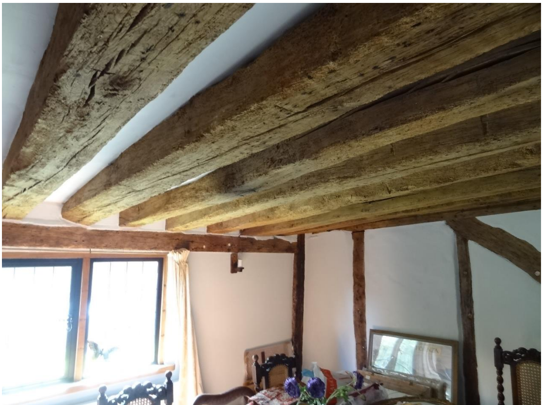
South side of old house – note flat joists, also elsewhere in the old house.
